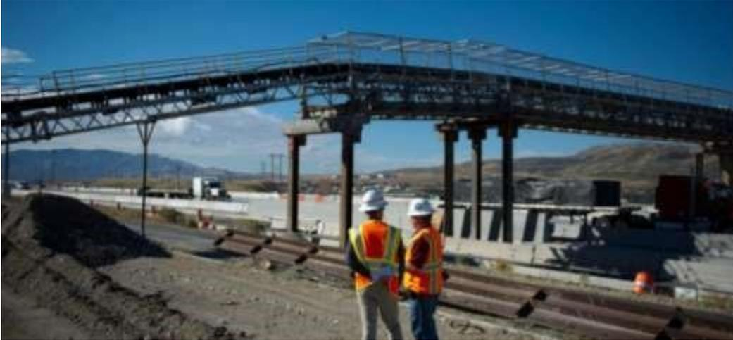
**Figure 1.** Section of a conveyer bridge overpassing a highway (screenshot from promotional material).
